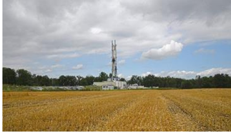
Photo 1 Polling drilling site.
