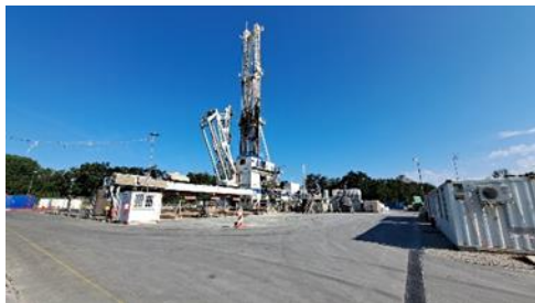
Photo 3 Polling drilling site.
