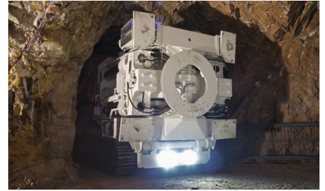
Vertical and inclined boreholes in confined spaces.
