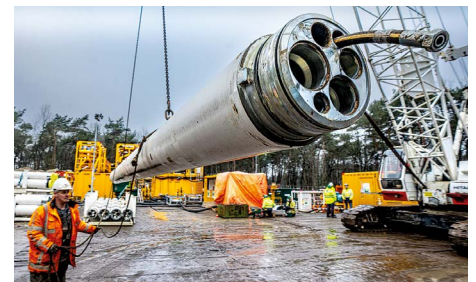
Steel pipes for continuous advance
