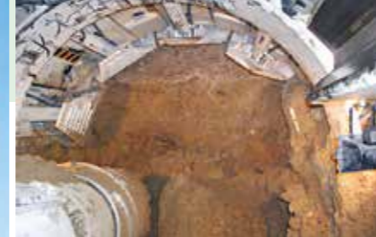
Front view of tunnelface during excavation.
