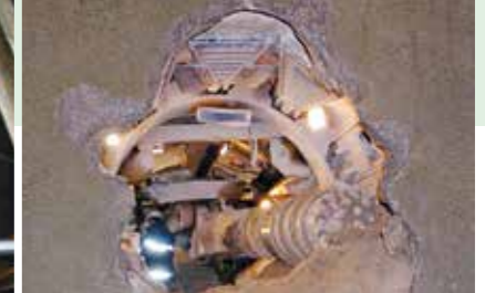
Breakthrough of MHSM2 Roadheader.
