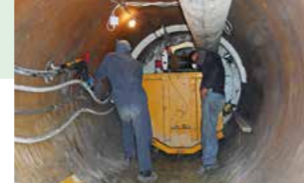
Pushing steel pipes.
