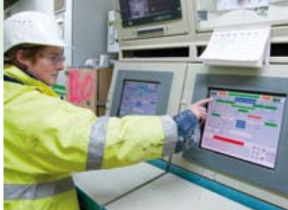
Computer-supported control and visualization in the control cabin of the separation plant.
