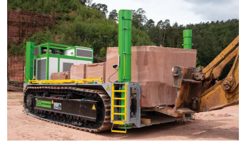
Unloading with conventional equipment.
